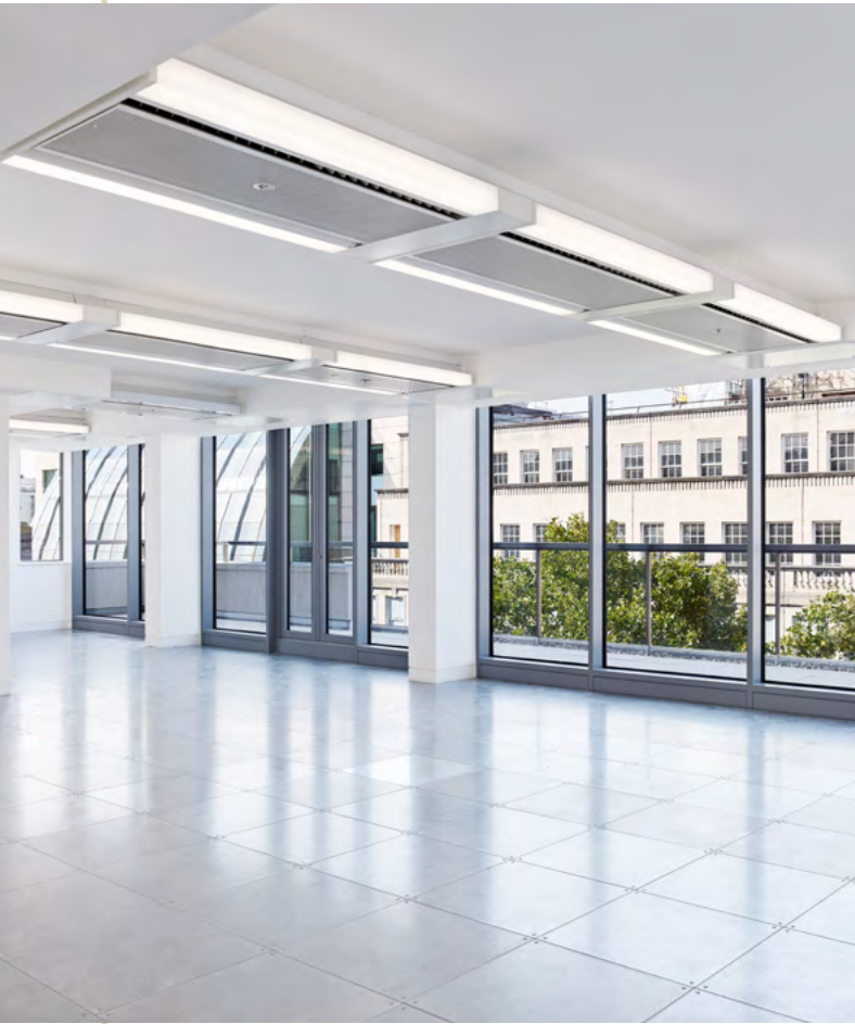
262 High Holborn Active Multi-Service Chilled Beams
