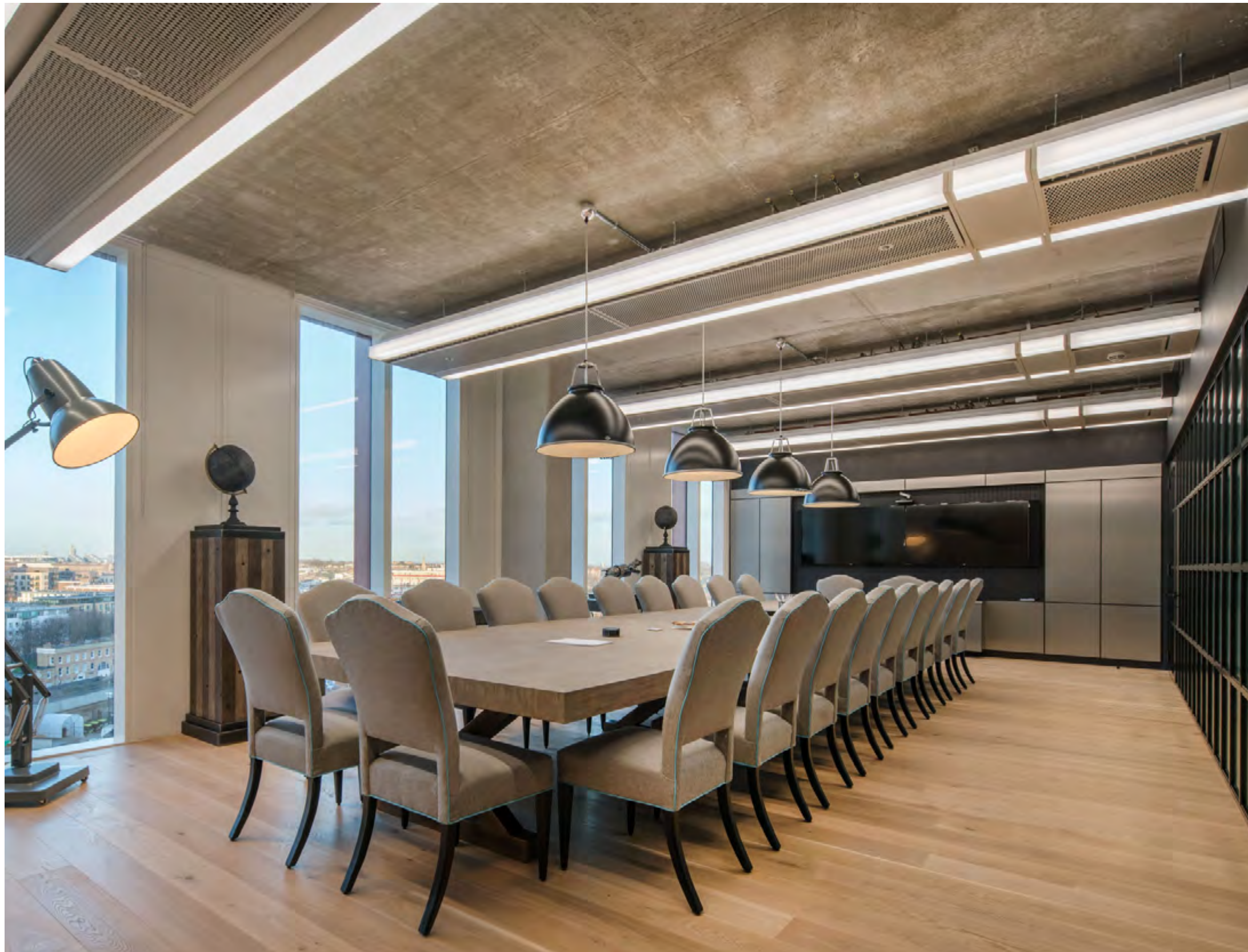
active multiservice chilled beams
