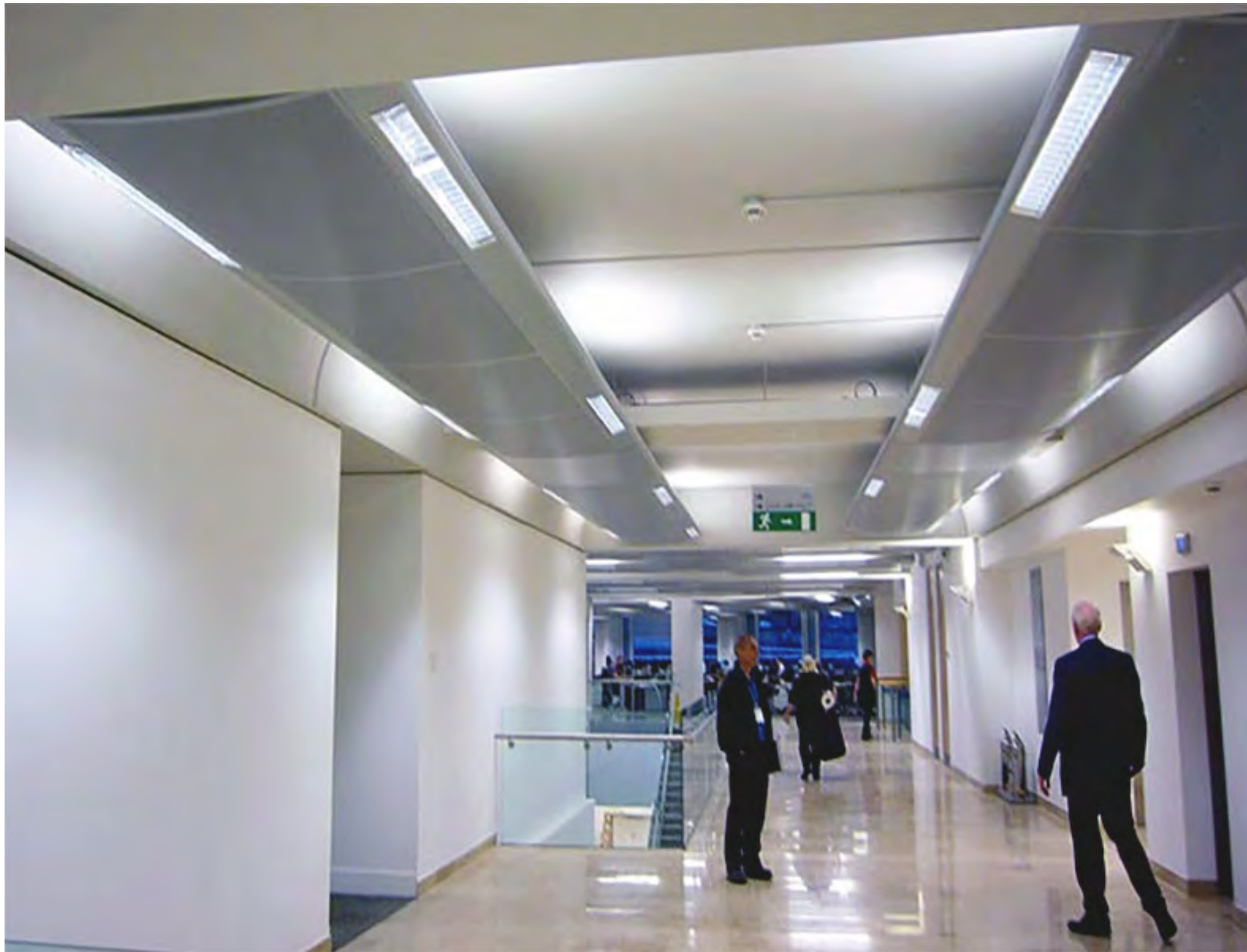
radiant passive multiservice chilled beams
