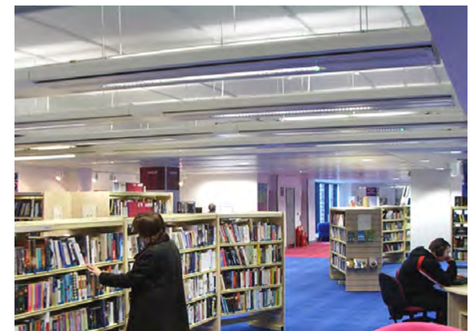
active multiservice chilled beams
