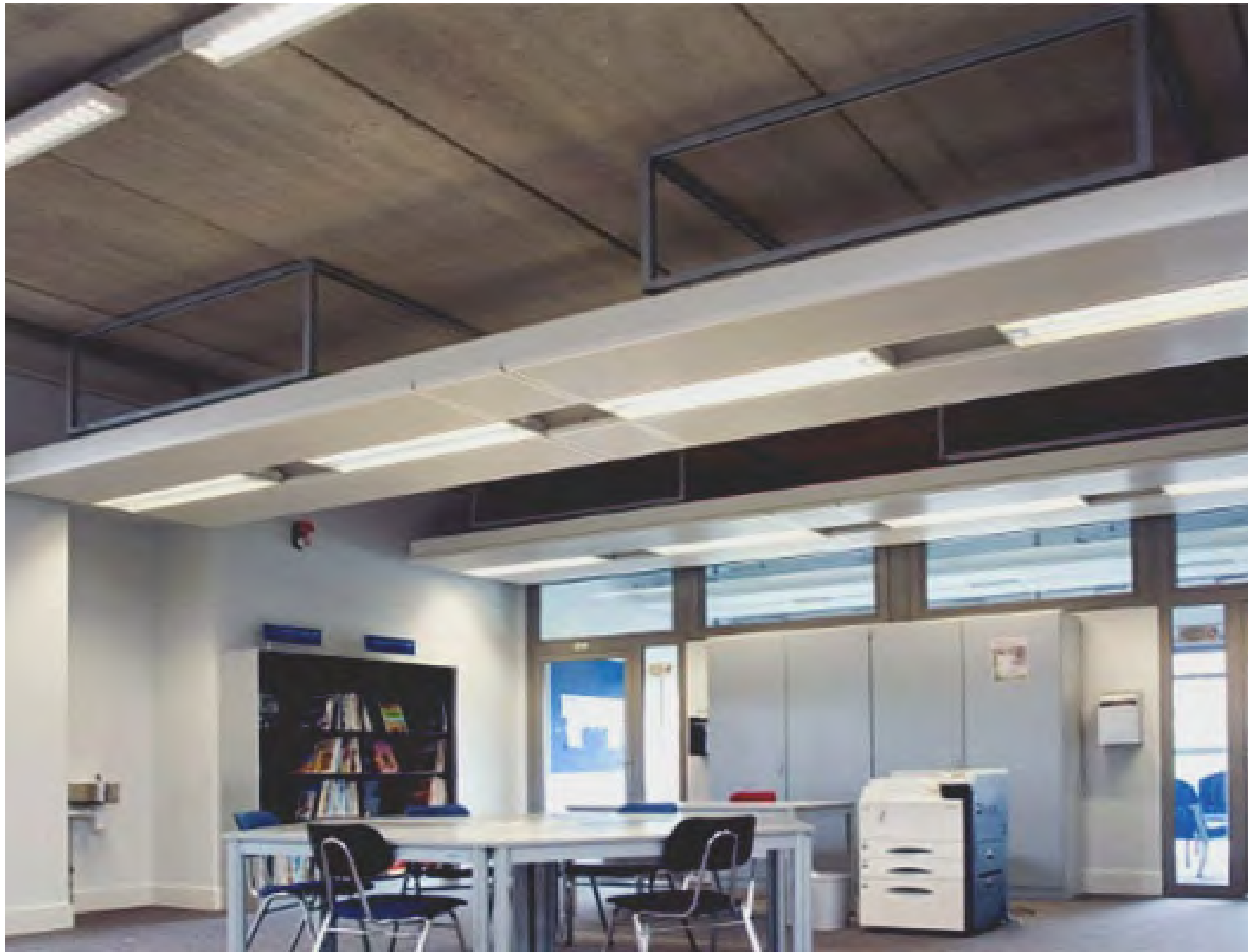
radiant passive multiservice chilled beam
