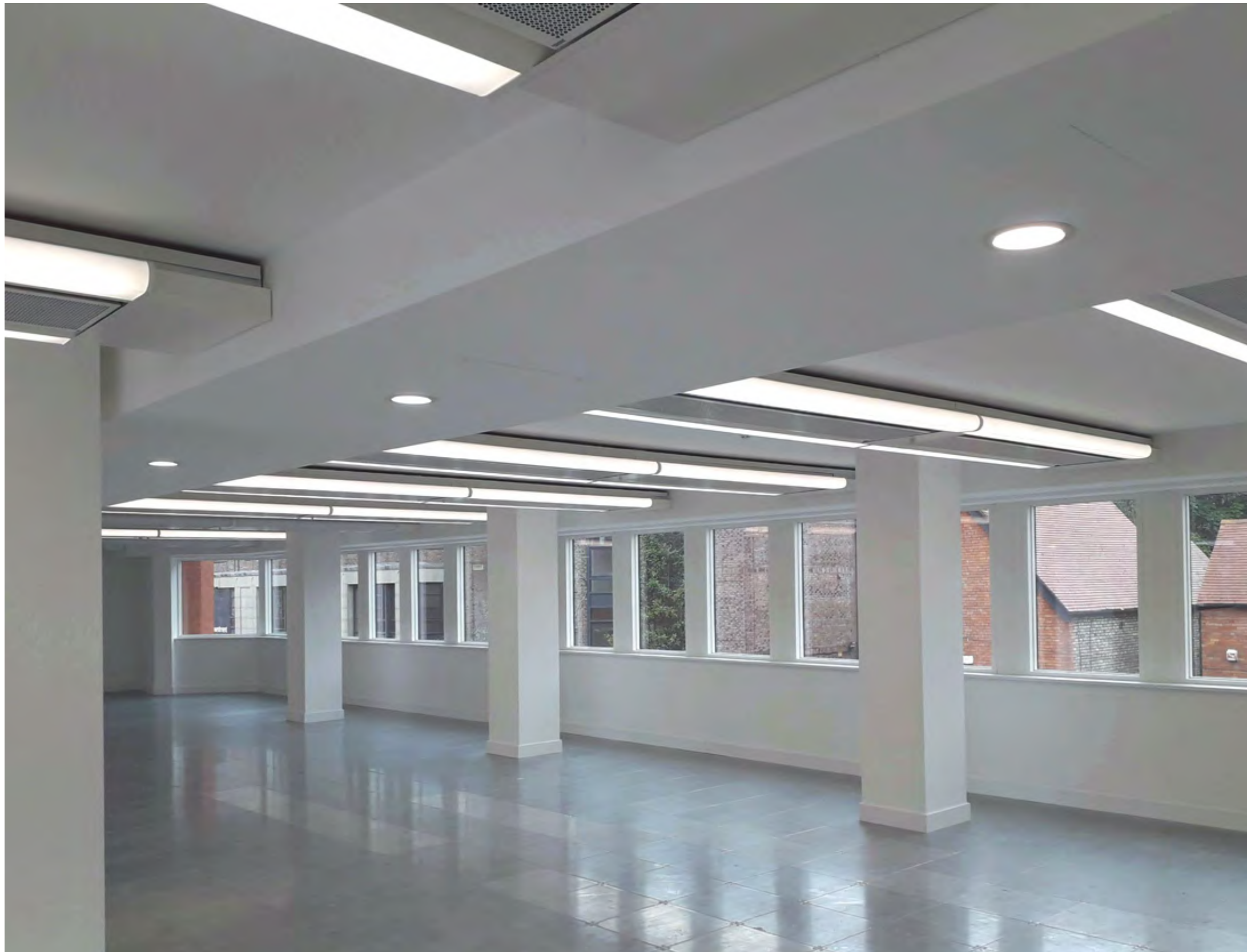
active multiservice chilled beams
