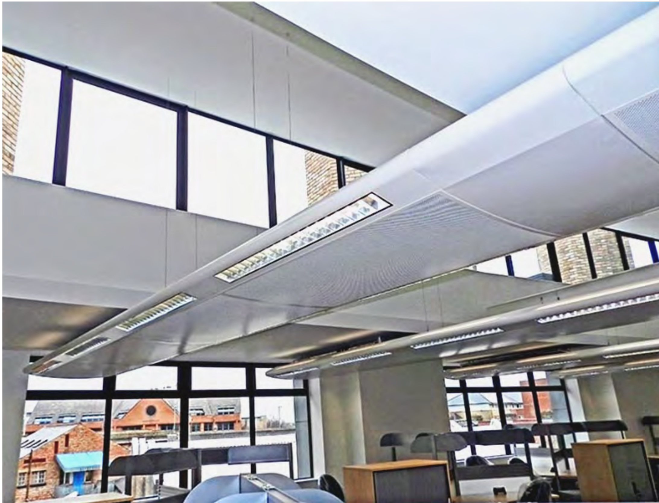
radiant passive multiservice chilled beams
