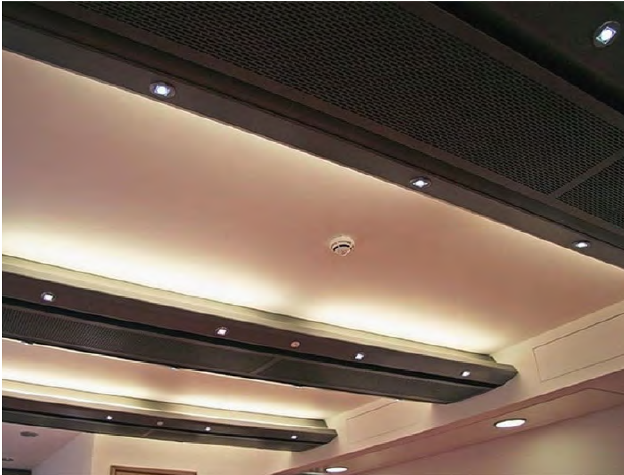
active multiservice chilled beams
