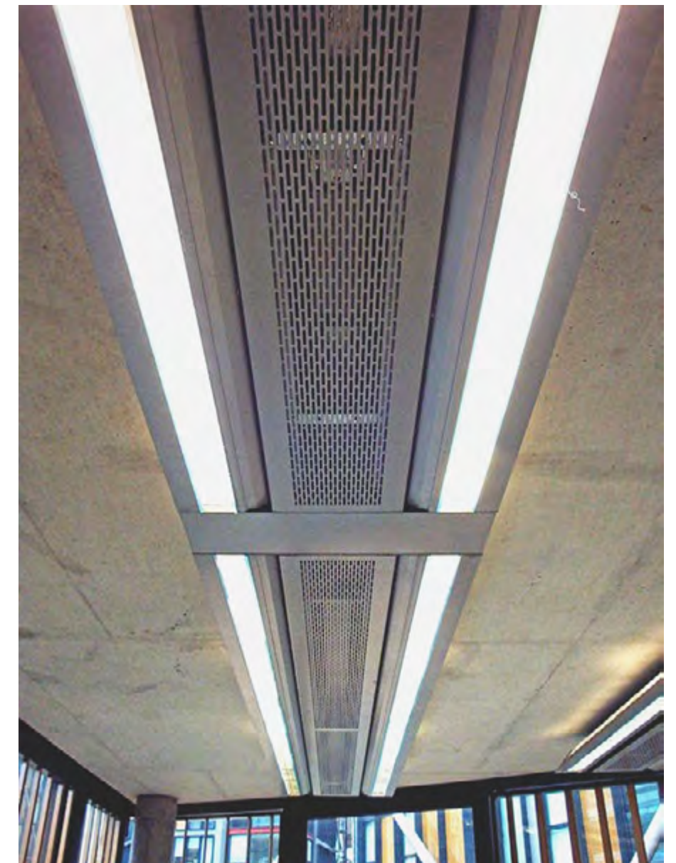
active multiservice chilled beams
