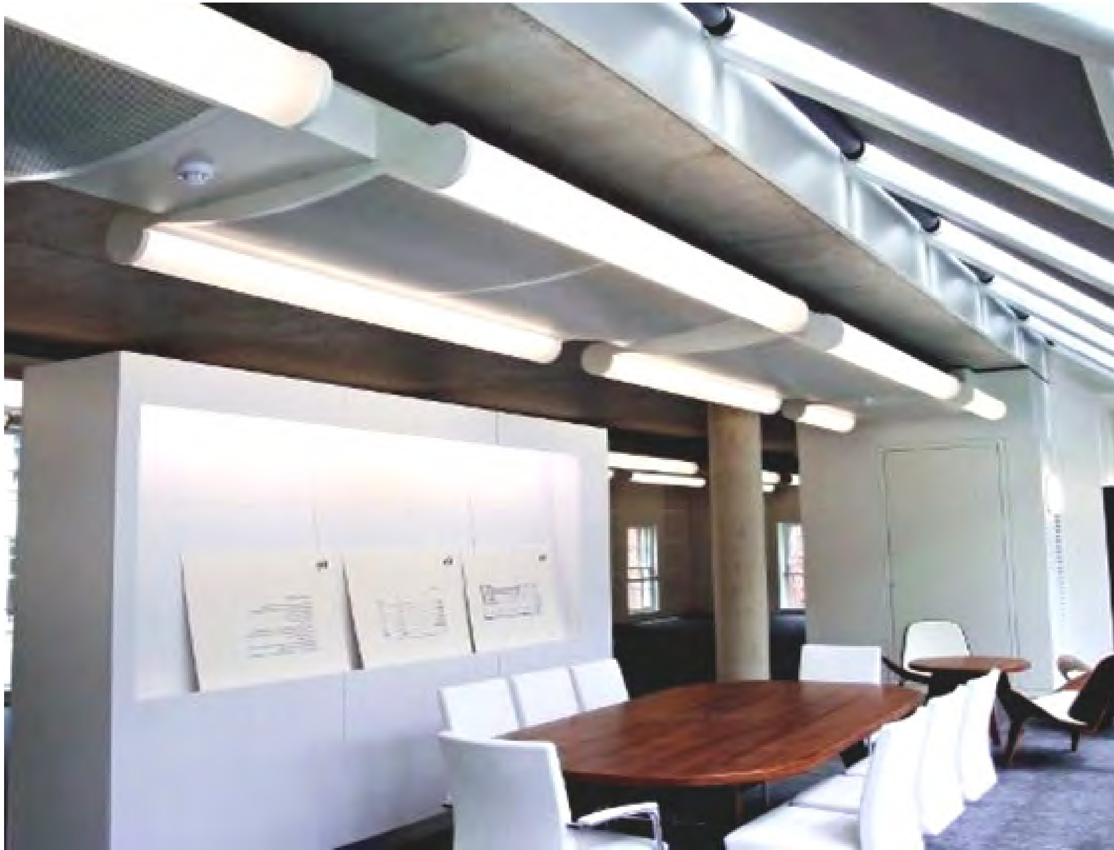
radiant passive multiservice chilled beams
