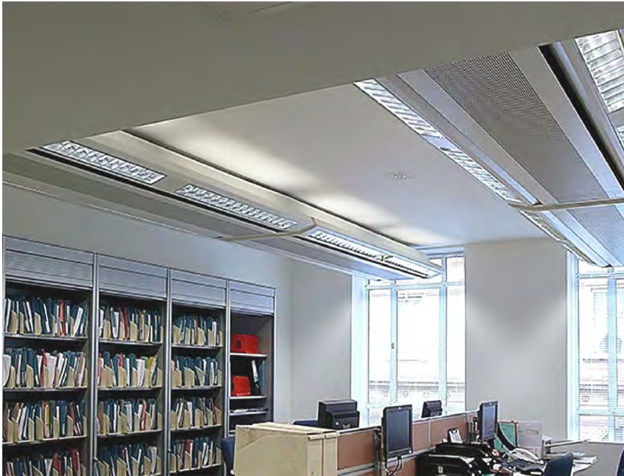
active ceiling integrated chilled beam
