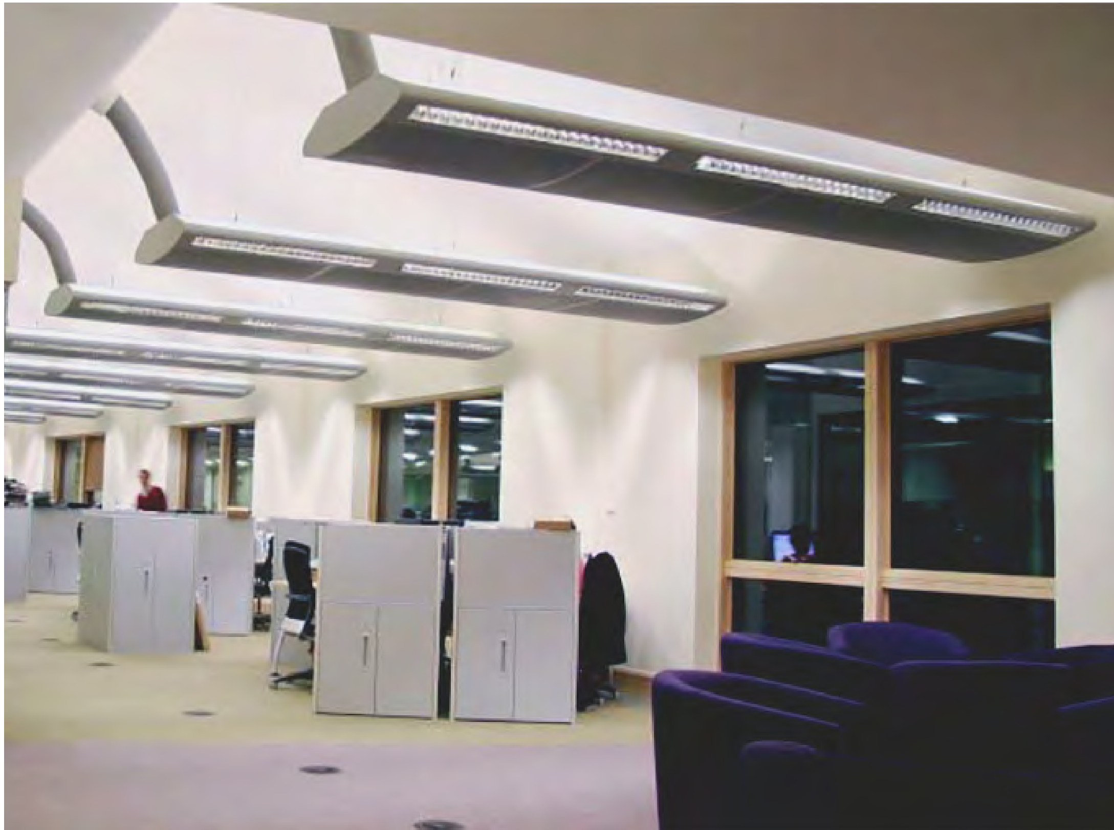
passive multiservice chilled beams, passive & active chilled beams
