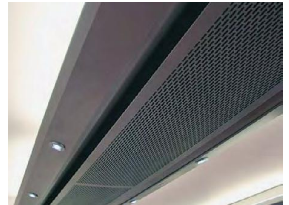
active multiservice chilled beams
