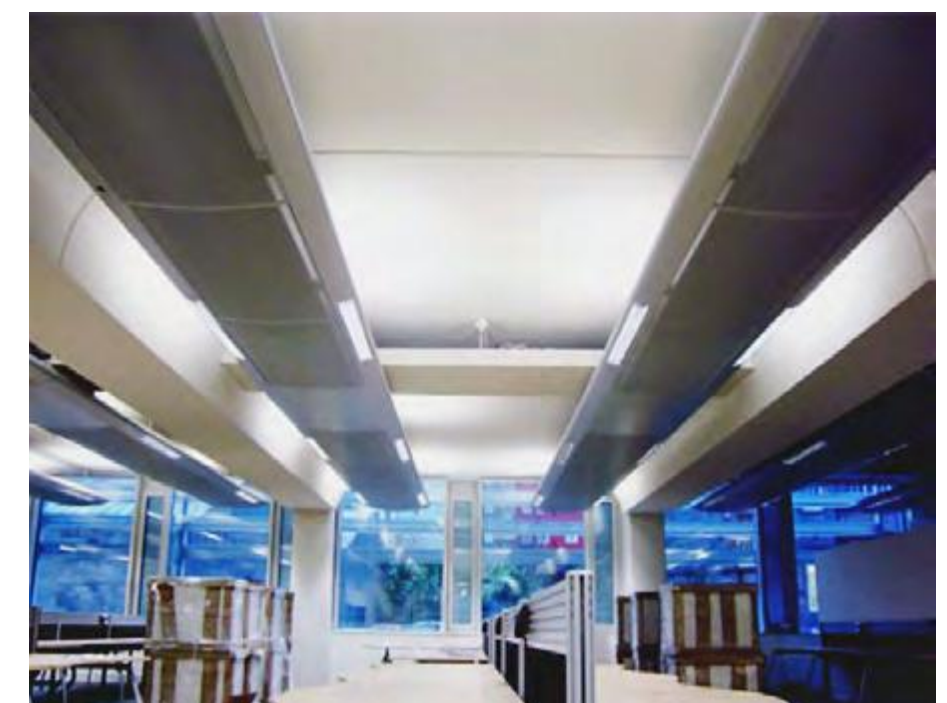
radiant passive multiservice chilled beams
