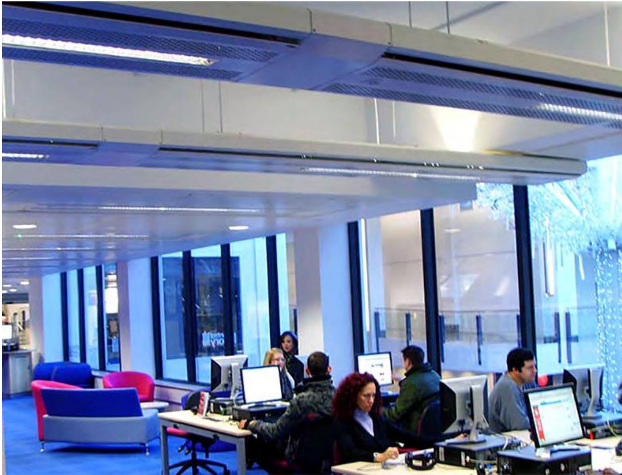
active multiservice chilled beams
