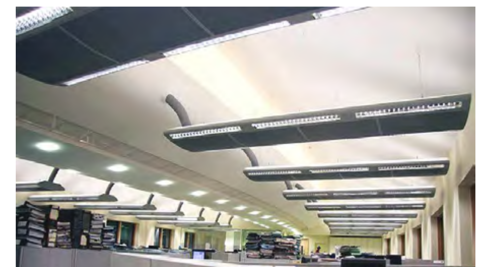
passive multiservice chilled beams, passive & active chilled beams
