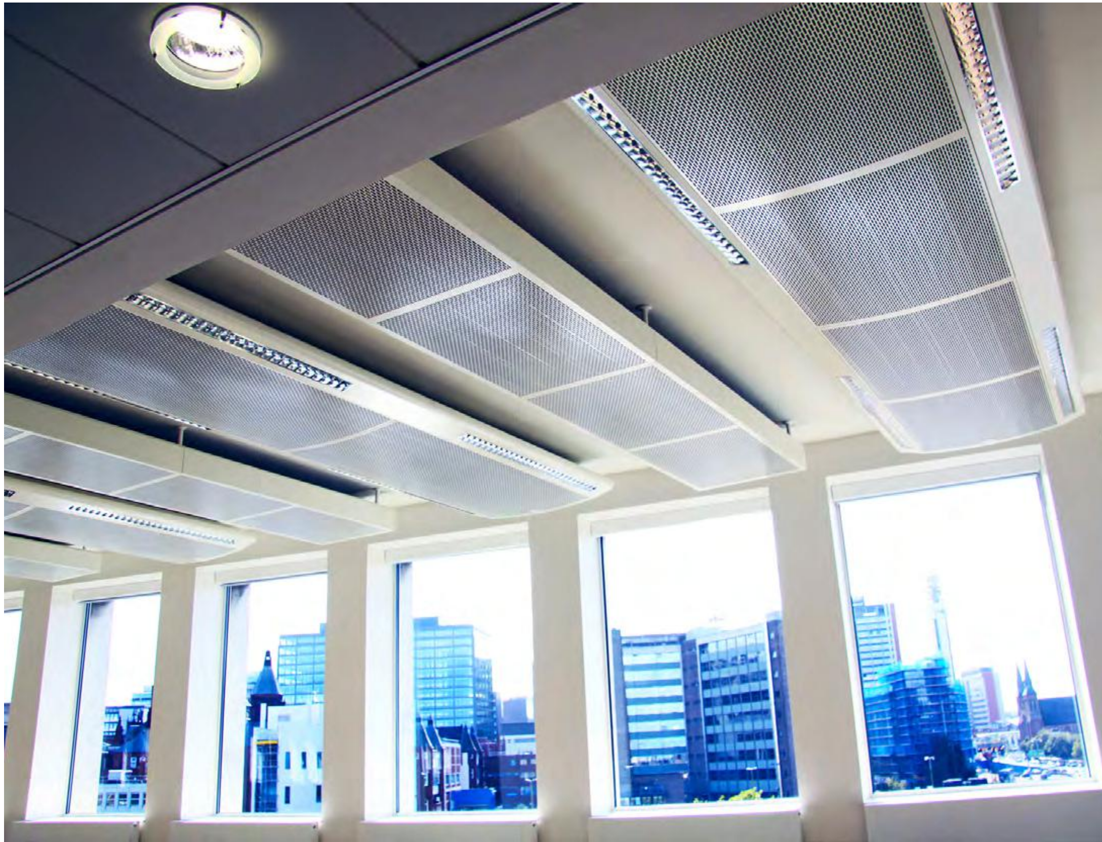
radiant passive multiservice chilled beam
