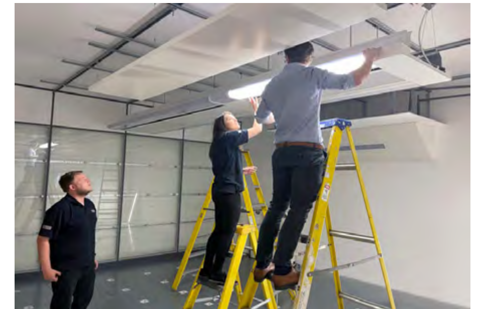
active multiservice chilled beams
