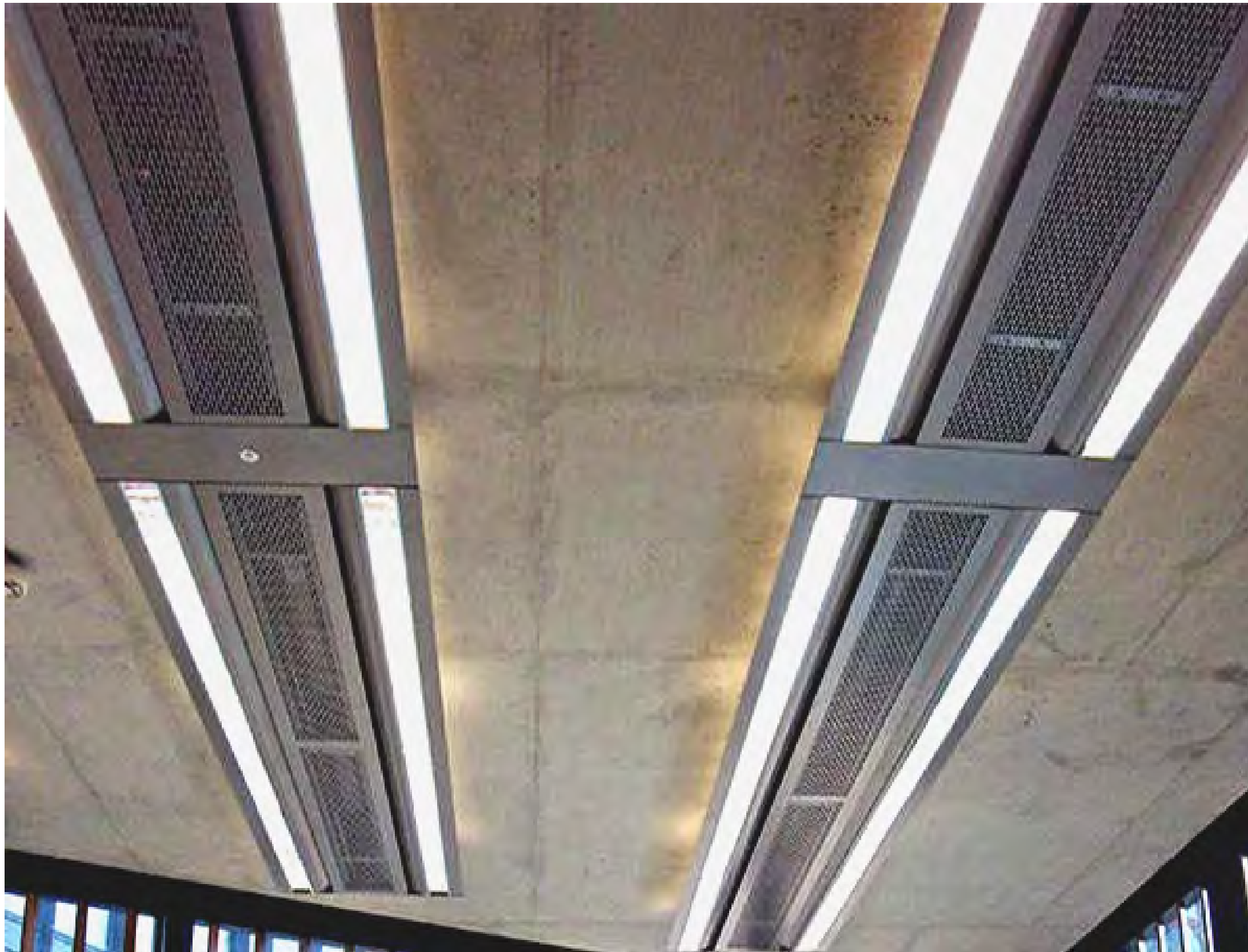
active multiservice chilled beams
