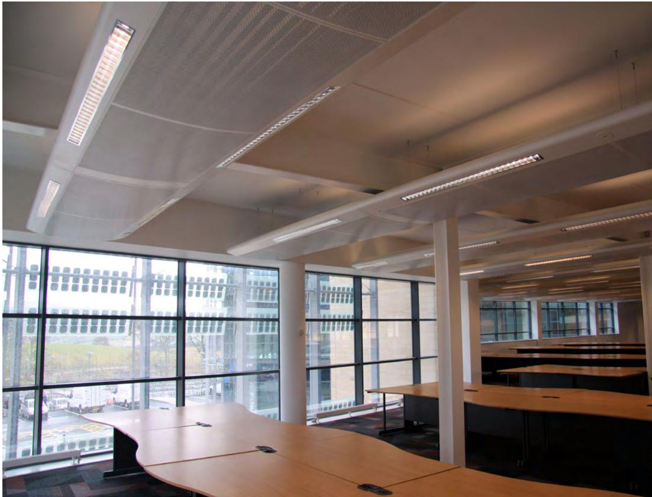
radiant passive multiservice chilled beams
