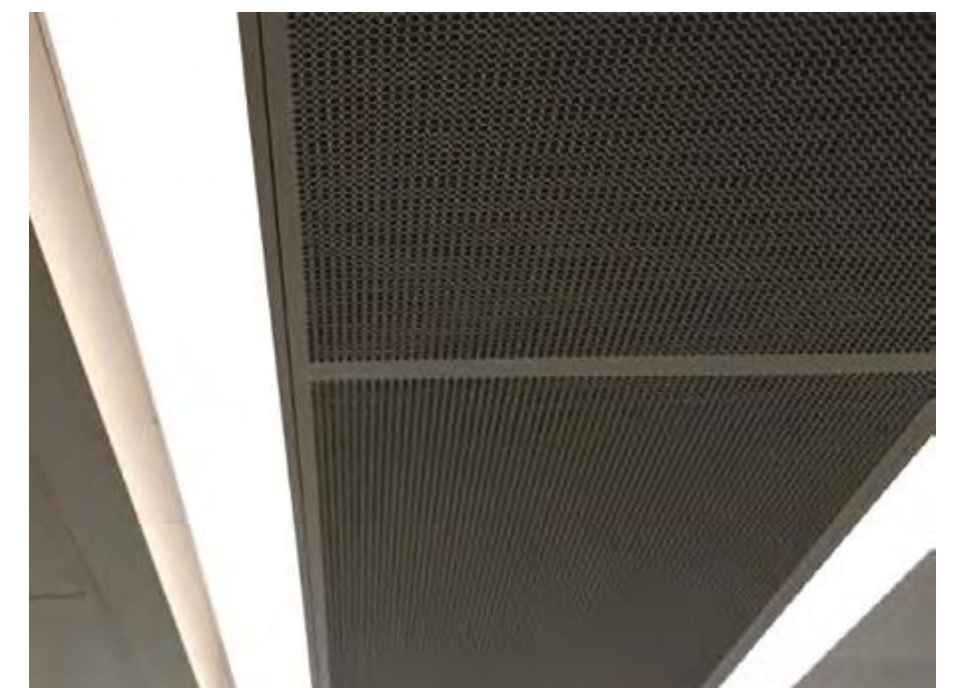
passive multiservice chilled beams
