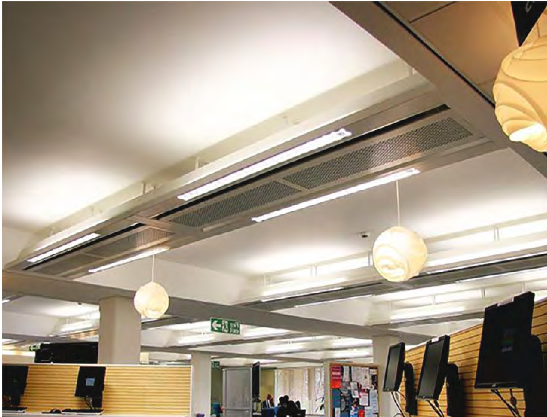
radiant passive multiservice chilled beams
