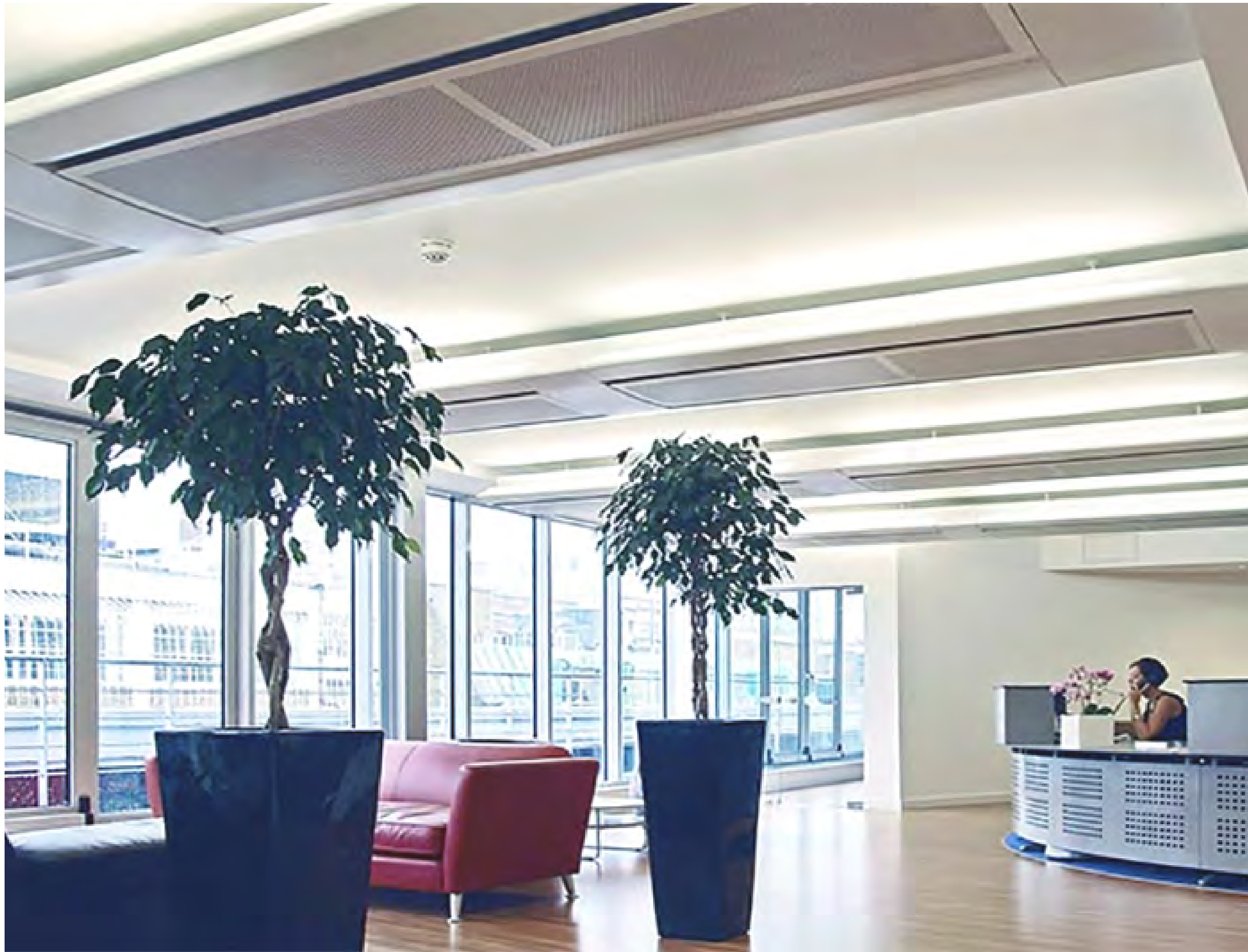
active ceiling integrated chilled beam
