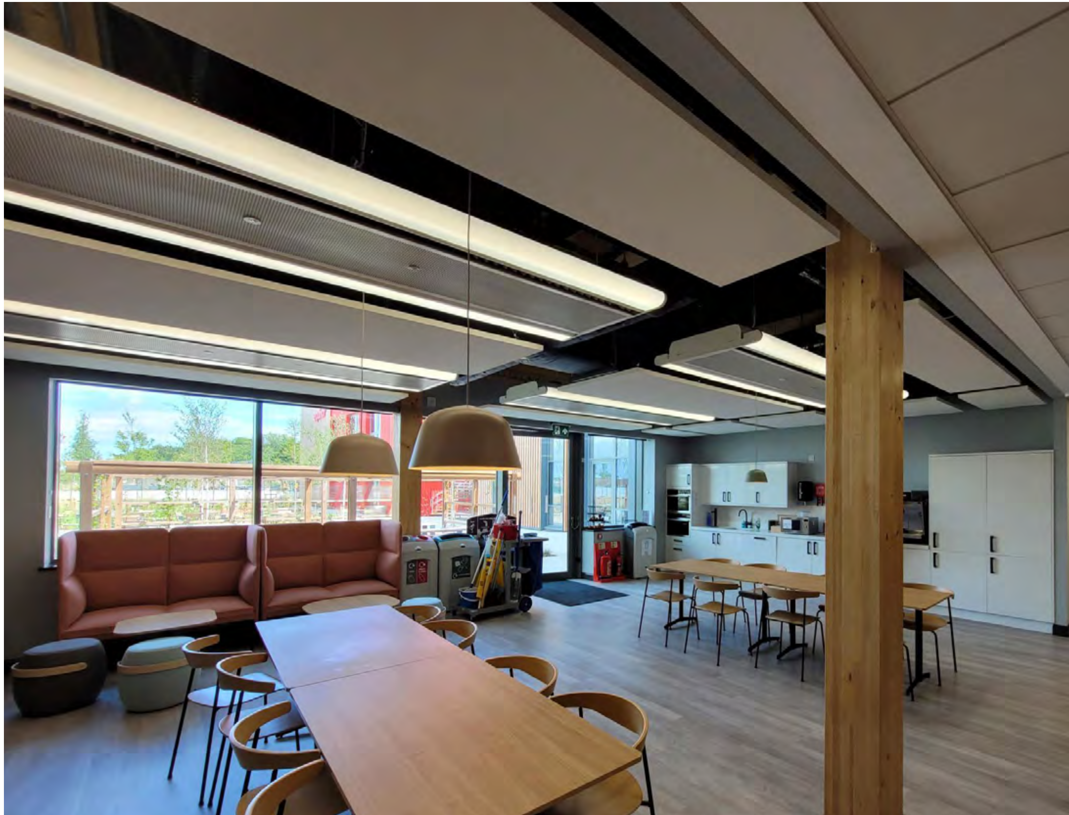
active multiservice chilled beams
